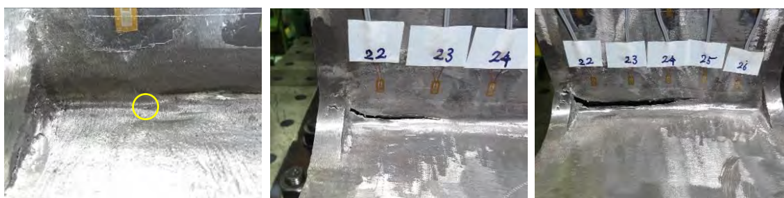
(a) 5 Half Cycle 載荷後 (b) 11 Half Cycle 載荷後 (c) 15 Half Cycle 載荷後
